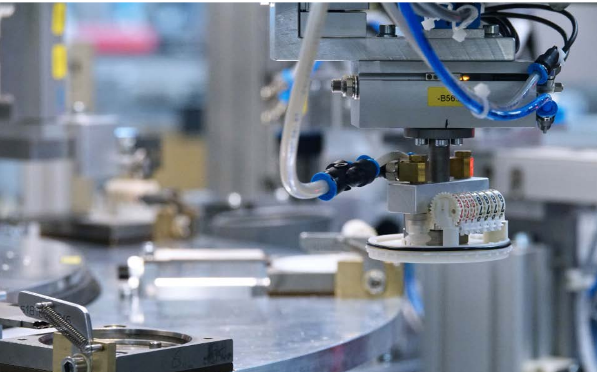
› Successful installation with a “double bottom:” The company subsidiary REX Automatisierungstechnik replaced the control system of a water meter testing system that had already been in use for 26 years. When testing the electrical equipment, including the control technology, the REX AT team ensured that it was possible to switch over to the existing, old system during trial operation of the installation.
