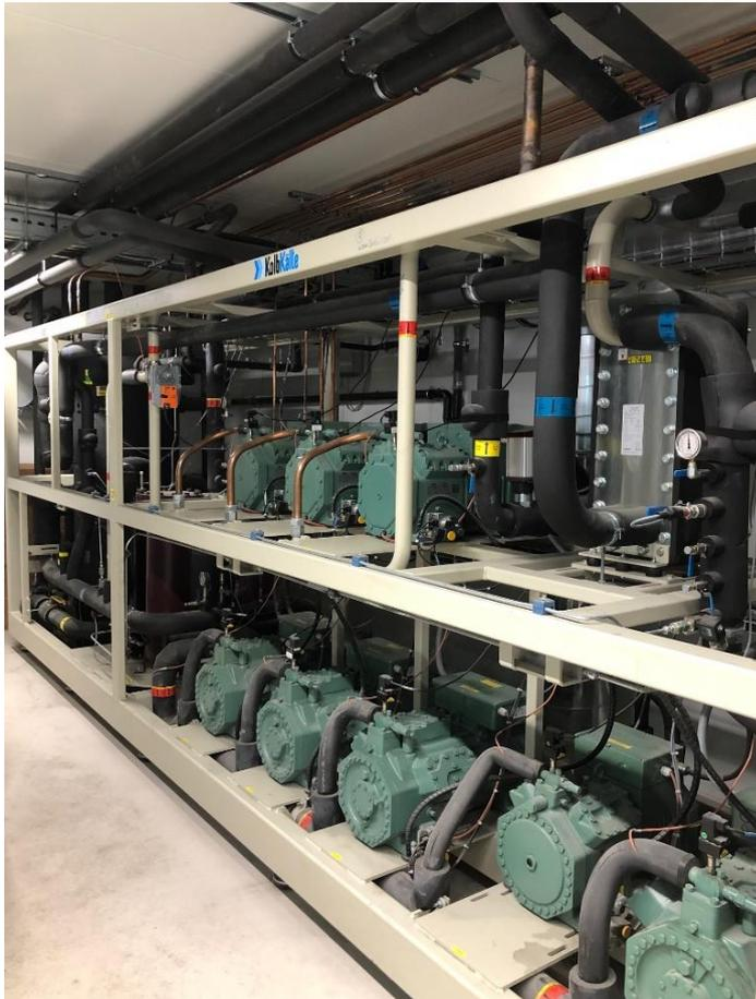
Fig. 3: The transcritical CO<sub>2</sub> booster system containing a total of 11 compressors (Photo: KOLB KÄLTE)
