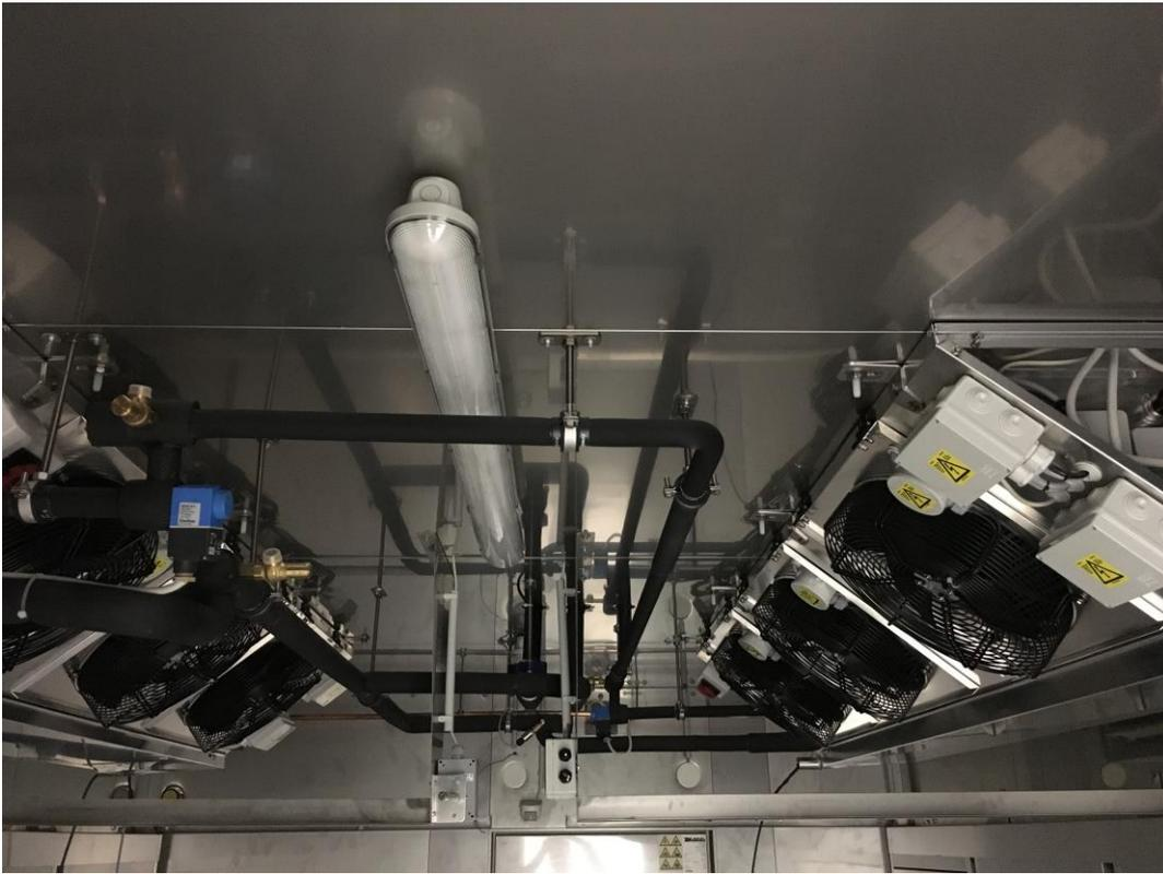
Fig. 5: Evaporators inside the fermentation interrupters (Photo: KOLB KÄLTE)
