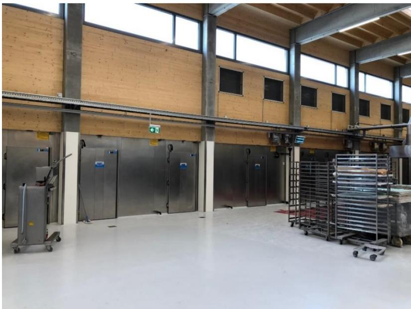
Fig. 1: The new facility has around 420 m<sup>2</sup> refrigerated space (a cooling capacity of 2580 m<sup>3</sup>) with a large number of refrigeration and freezing rooms as well as temperature-controlled rooms for fermentation. (Photo: KOLB KÄLTE)
